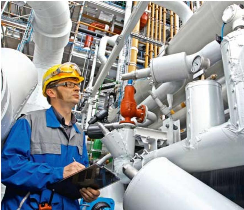
Gas circulation system for polysilicon production at the plant in Nünchritz. Resulting by-products are recycled in the system to be added back into the manufacturing process.
